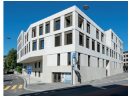
Altstätten Churerstrasse 1a, 1b, 1c
