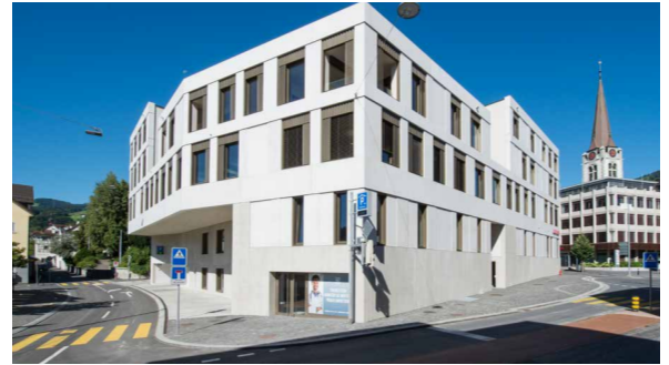
Altstätten, Churerstrasse 1a, 1b, 1c
